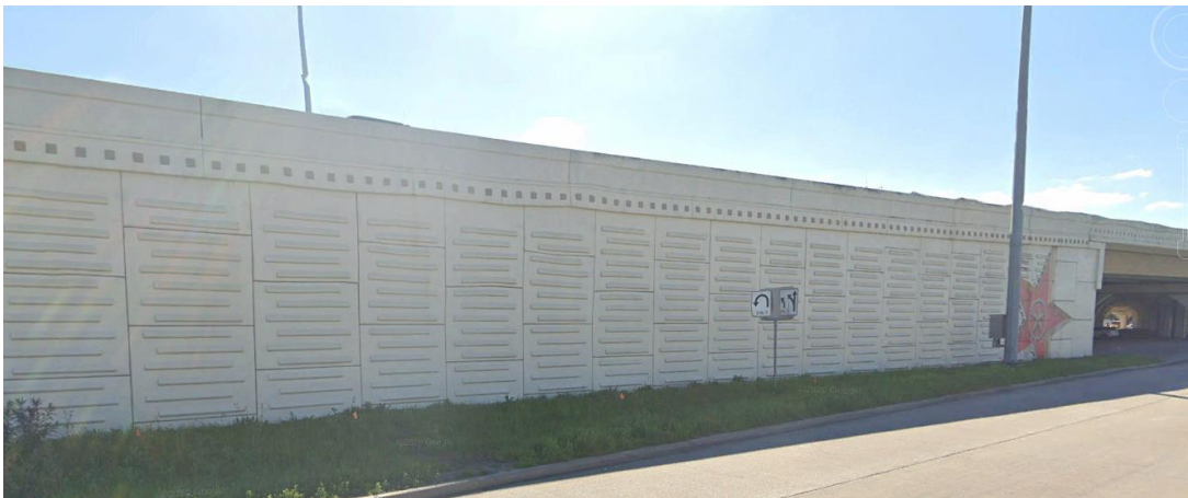
MSE Retaining Wall: I-10 @ Katy Fort Bend Rd (Katy)
