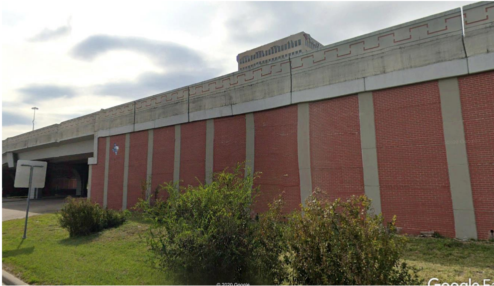
MSE Retaining Wall: IH 610 @ Bissonnet St (Houston)
