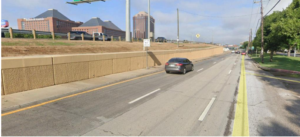
MSE Retaining Wall: I-35E @ Market Center Blvd (Dallas)
